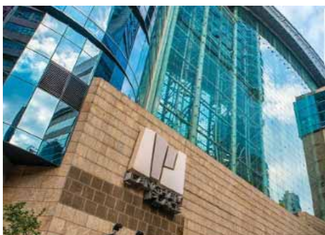
“LANGHAM PLACE” Address: 8 Argyle Street, Mongkok, Kowloon, Hong Kong
